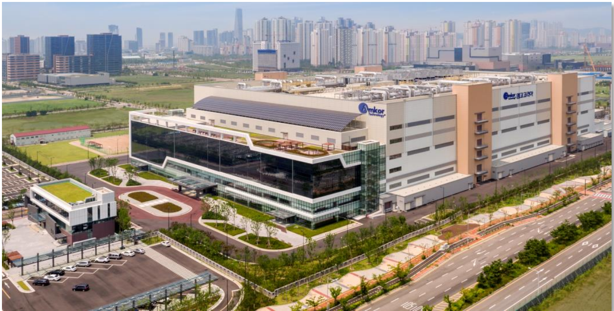
Figure 10. Example of an ATP facility
